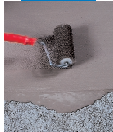
Using a roller on freshly applied Plano 3
