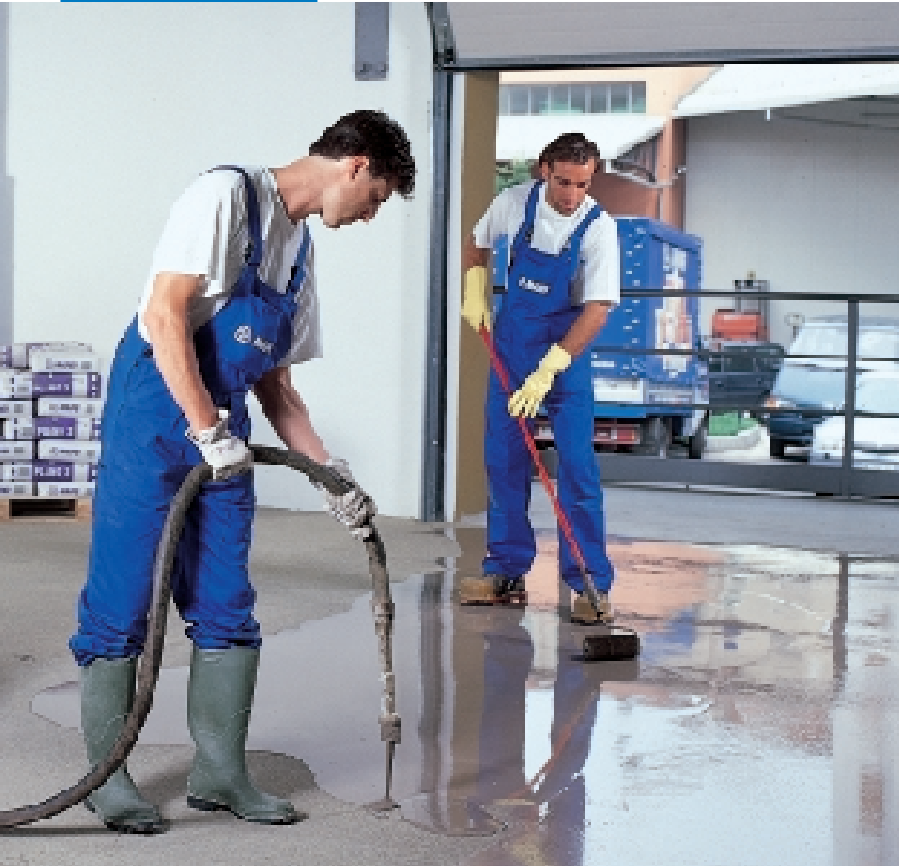
Applying Plano 3 with a pump
